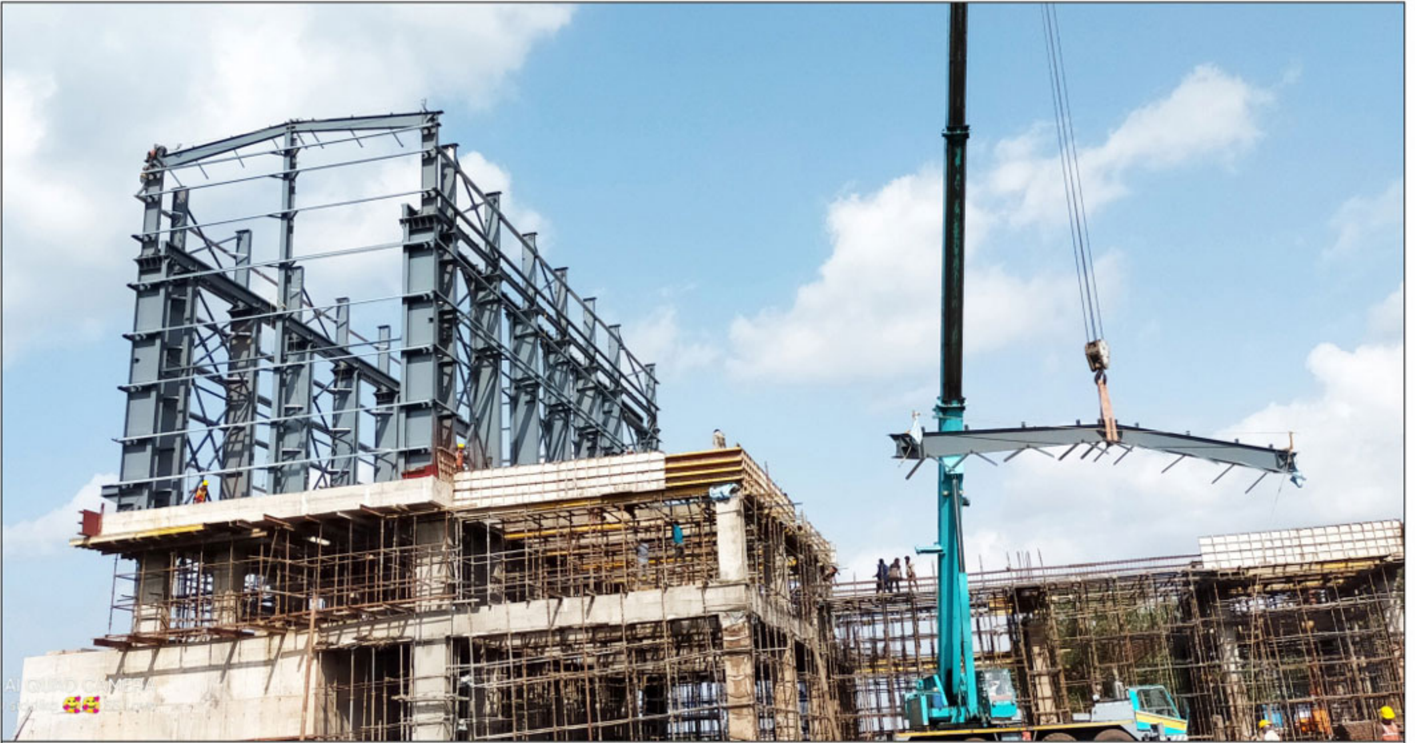
Pump House with 50 Mt Crane Facility
