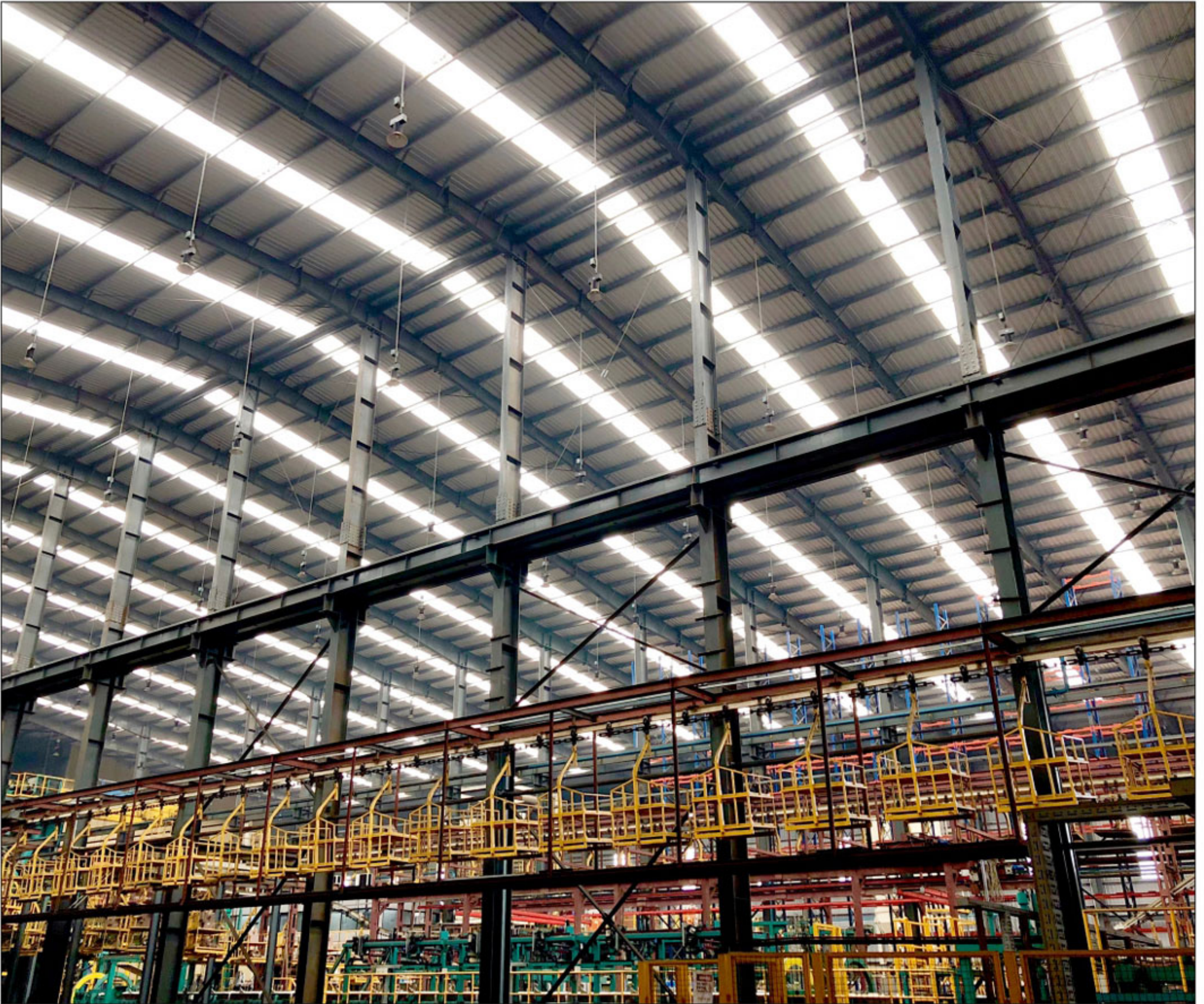
Foundry Processing Unit, Area : 1.0 Lakh Sq. Ft.
