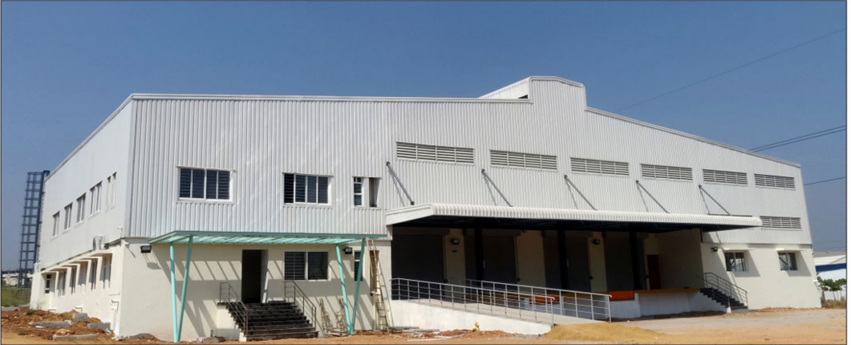
Tissue Manufacturing with Clear Span of 160'
