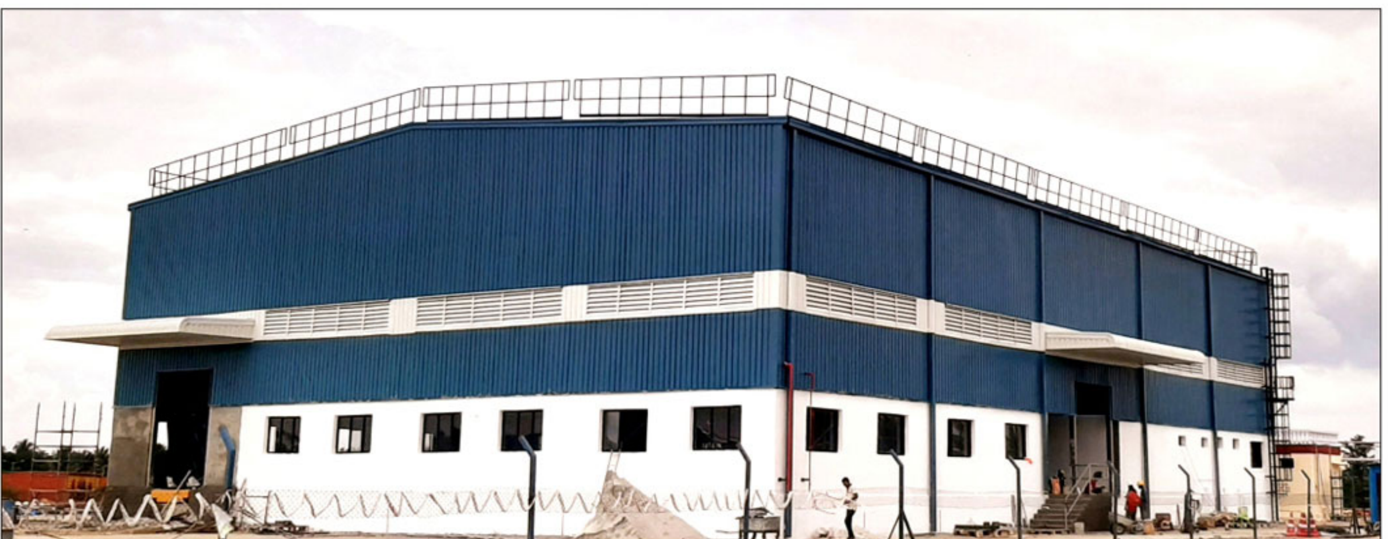
Paint Processing Unit
