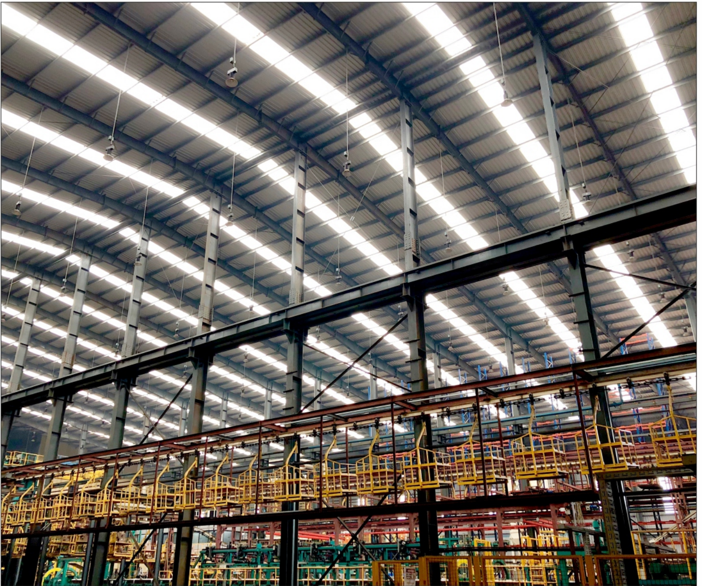
Foundry Processing Unit, Area : 1.0 Lakh Sq. Ft.
