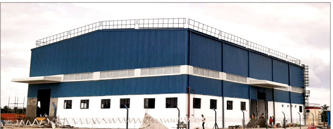
Paint Processing Unit
