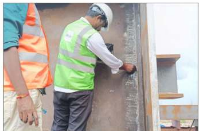
Ultrasonic weld test (UT)
