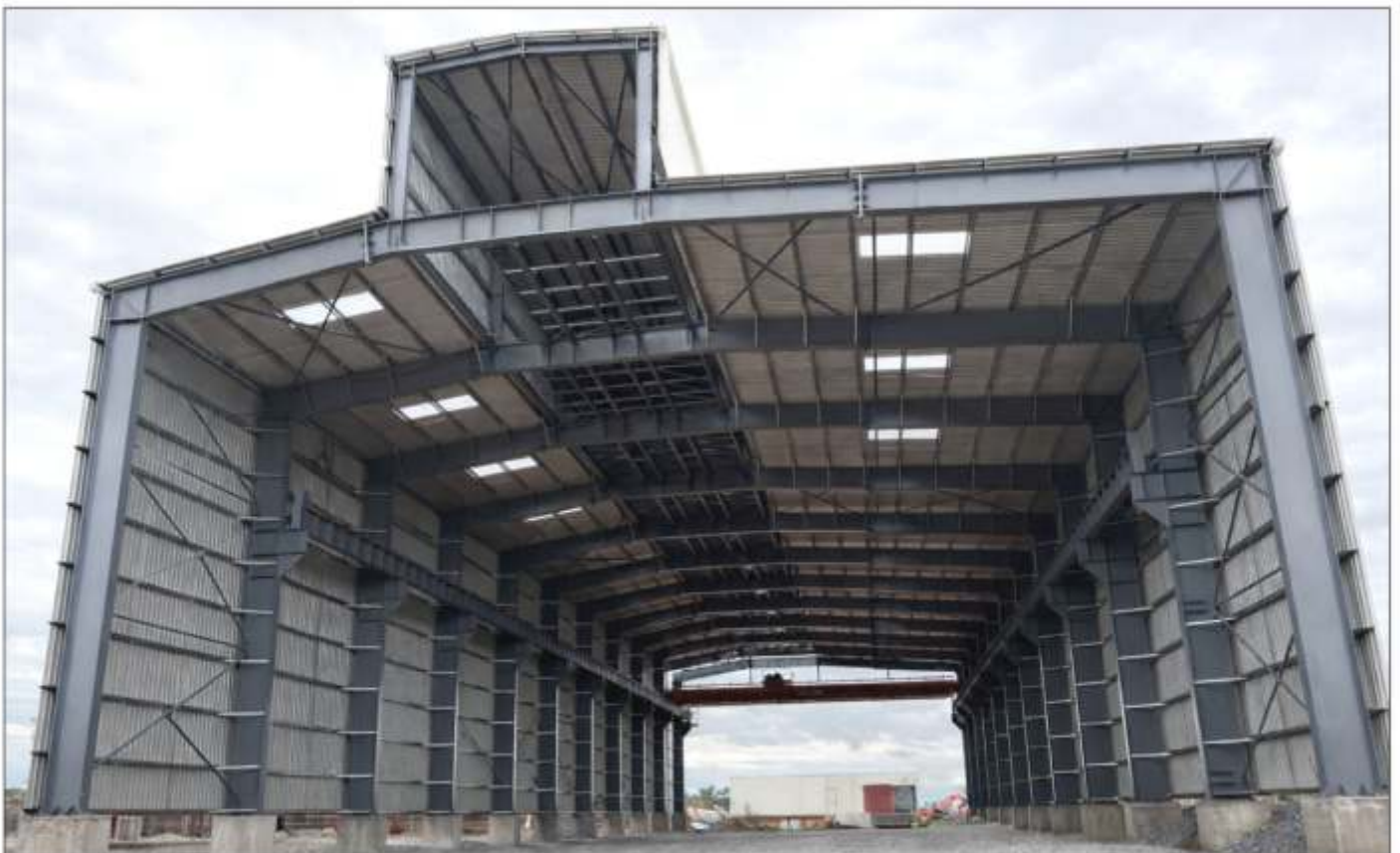
Concentrate Filter Cake Shed with 15 MT EOT crane and Conveyor system, Hospet.
