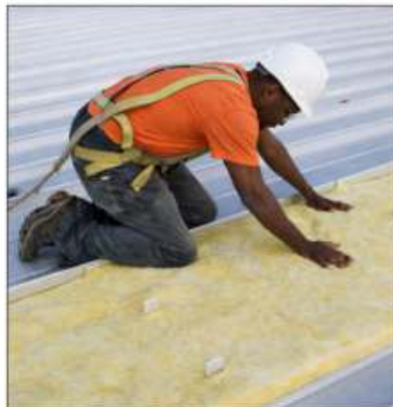
Insulation Laying
