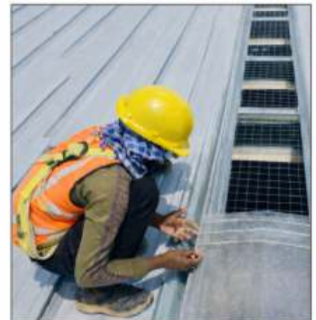
Polycarbonate Sheet Laying
